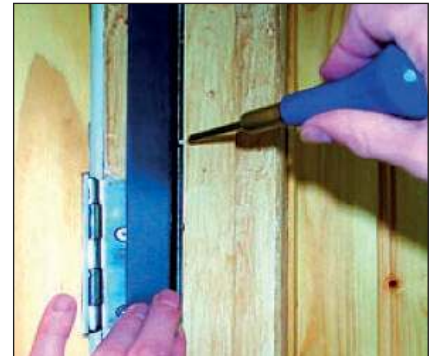
Step 3: Panel pins finish
